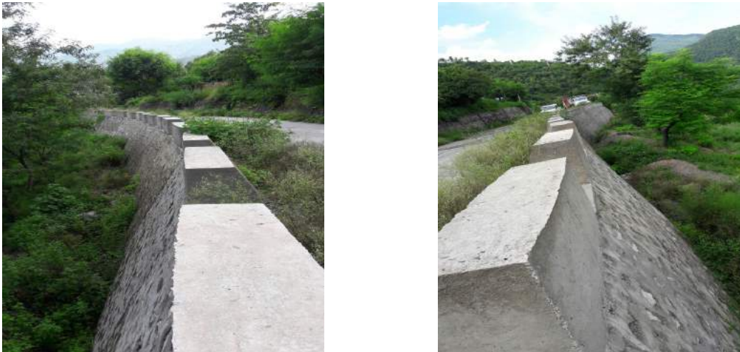
Protection Works at KHEP
