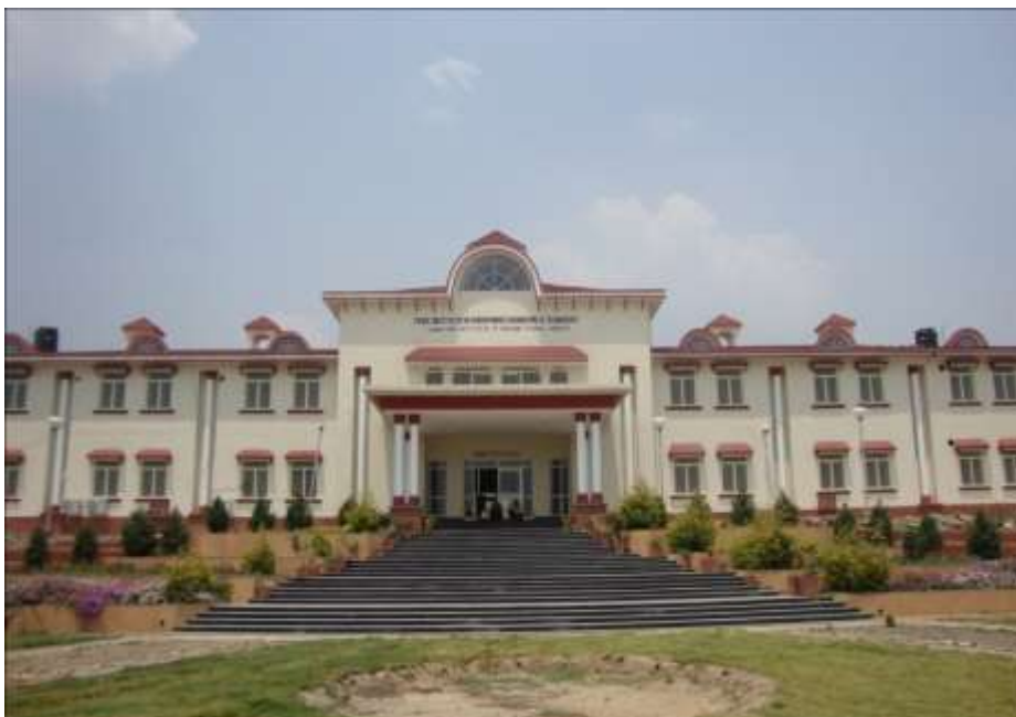
THDC Institute of Hydropower Engineering and Technology.
