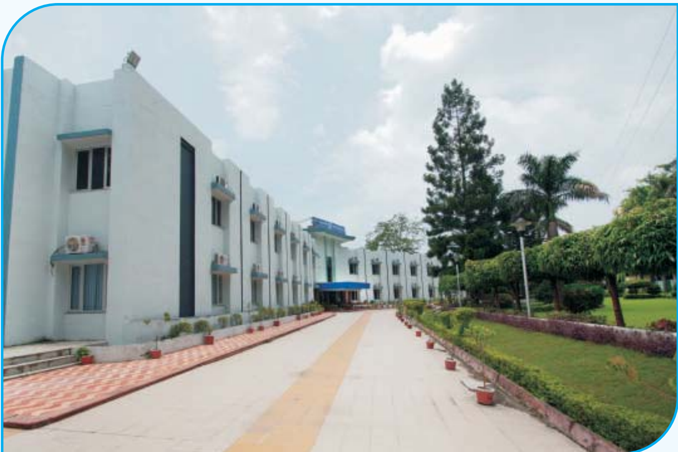
A view of Ganga Bhawan, THDCIL Corporate Office, Rishikesh
