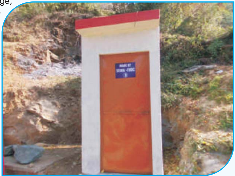
Individual Toilet constructed at Deen Gaon
