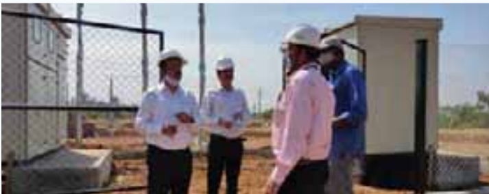
Visit of THDCIL Officials at the time of Commissioning of Project
