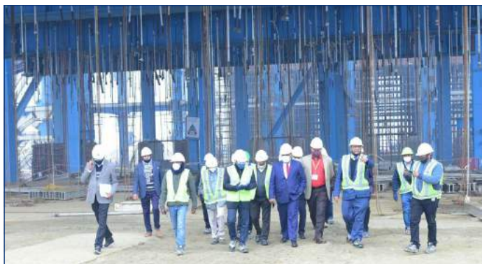
A view of the Commencement of Ceiling Girder of unit #1
