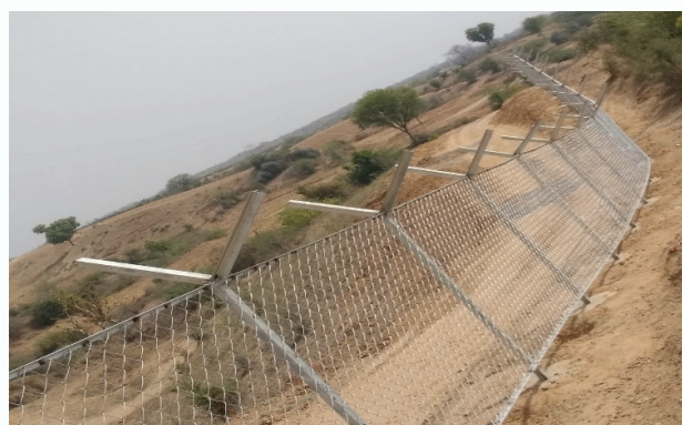
Fencing Work at Jhansi Solar Power Park
