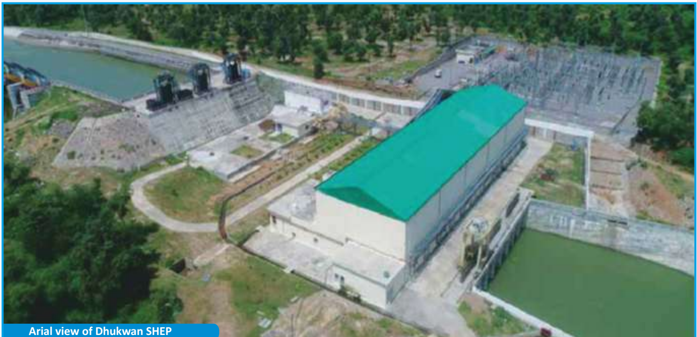
Aerial view of Dhukwan SHEP
