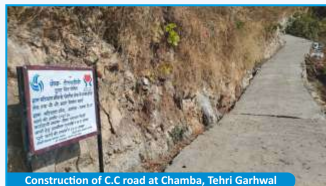
Construction of C.C road at Chamba, Tehri Garhwal
