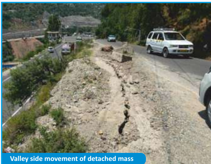
Initial subsidence observed on the Road
