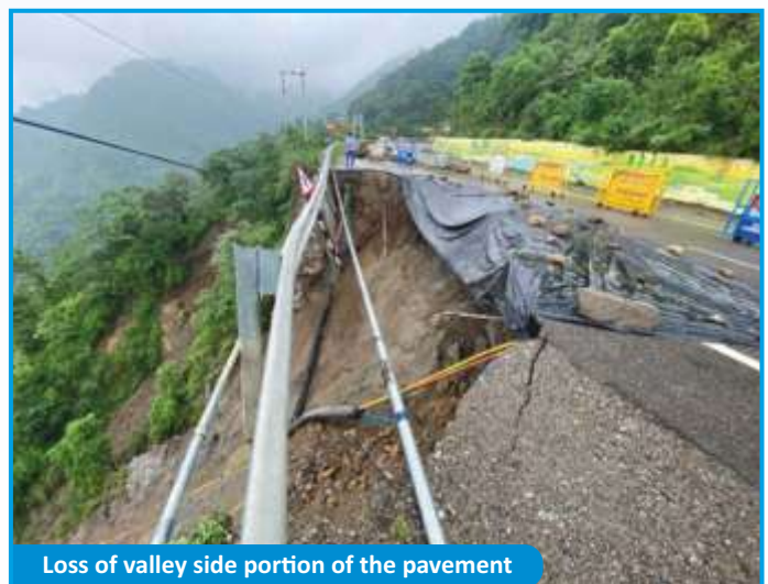
Prominent Cracks developed on the pavement
