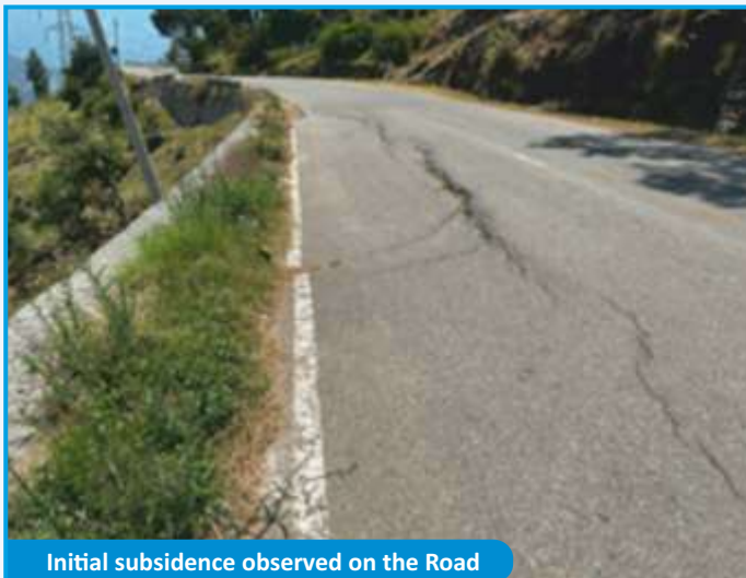
Prominent Cracks developed on the pavement
