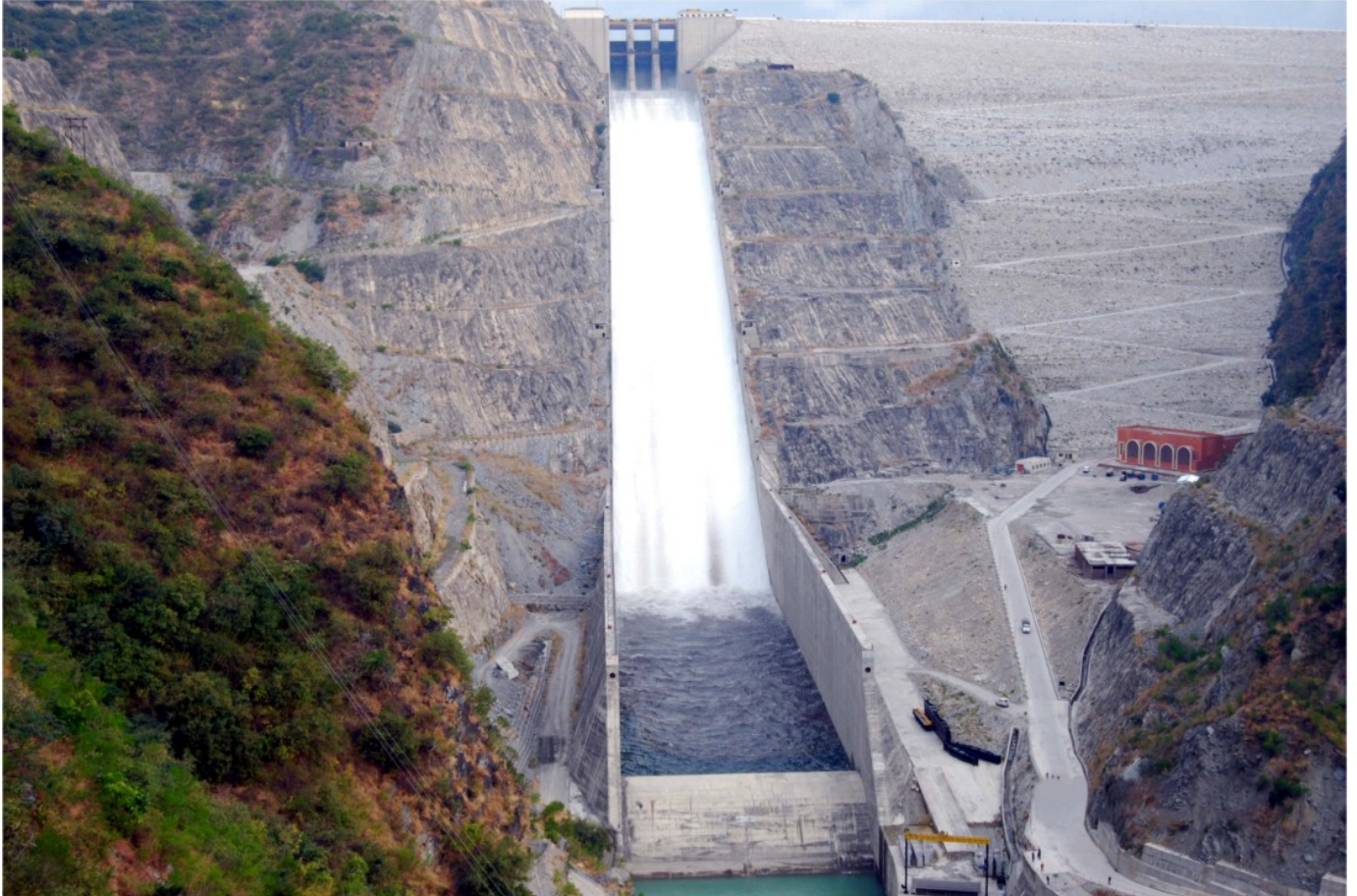
A view of Tehri Spillway
