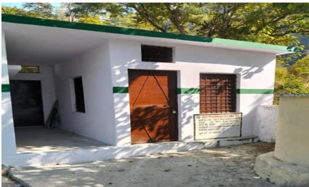
Fig: Construction of a kitchen at a Government Primary School in Village Chopra, District Tehri.
