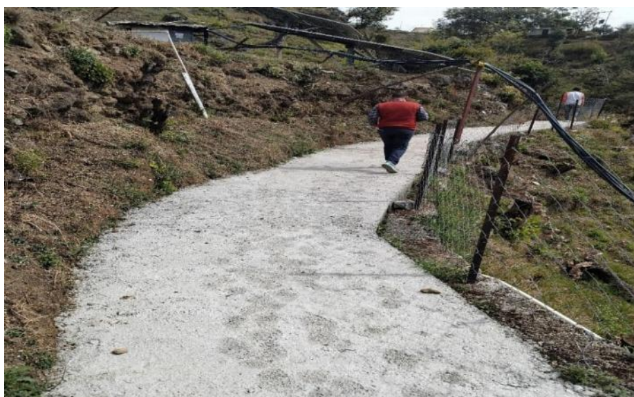
Fig: Constructed CC Road at GP Maithan Gaon, Tehri Garhwal, Uttarakhand
