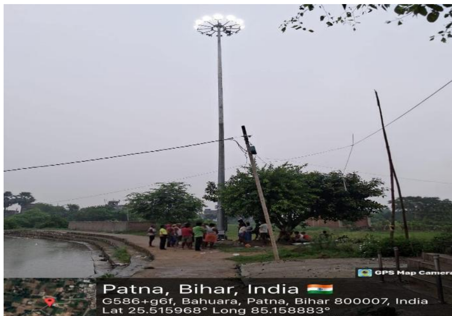
Fig: High mast lights were installed in villages, Patna, Bihar
