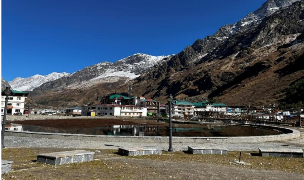
Fig: Construction of Lakefront at Badrish Lake & Park at Badrinath towns, Chamoli, Uttarakhand
