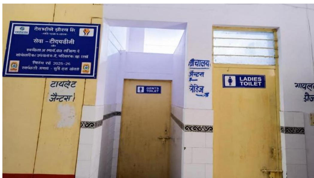
Fig: Renovation of Public Toilets at Tehsil Office Haridwar, Uttarakhand
