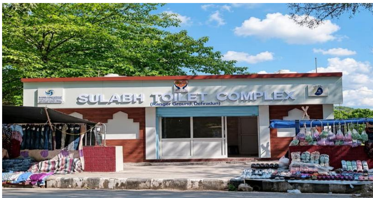
Fig: Construction of Public Toilet at Ranger Ground, Dehradun, Uttarakhand
