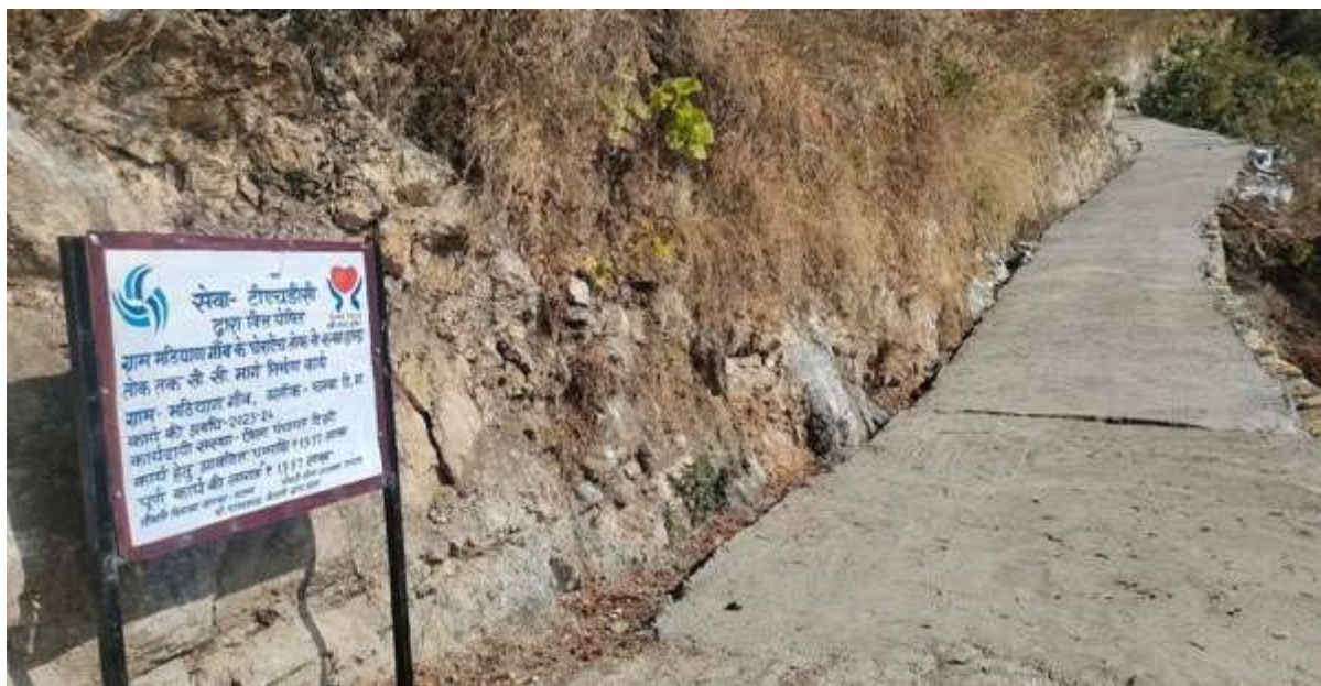
Fig: Construction of C.C road at Chamba, Tehri Garhwal
