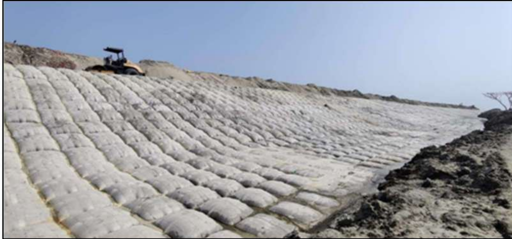
Fig. Image showing installed Articulating Grouted Concrete Mattress over canal slope protection
