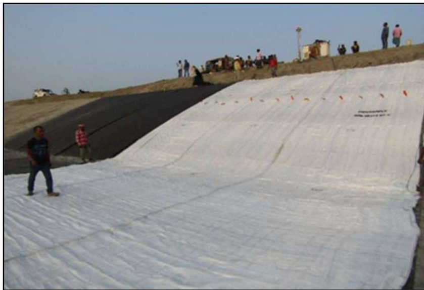
Fig. Laying of fabric
