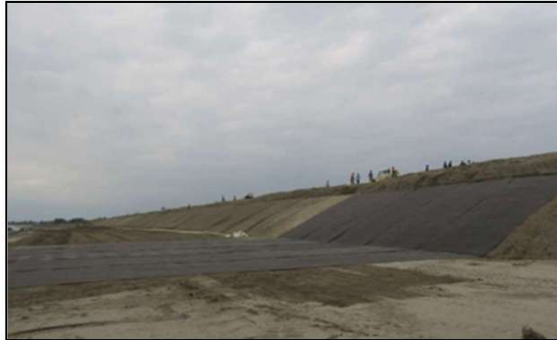
Fig. Laying of Geotextile layer
