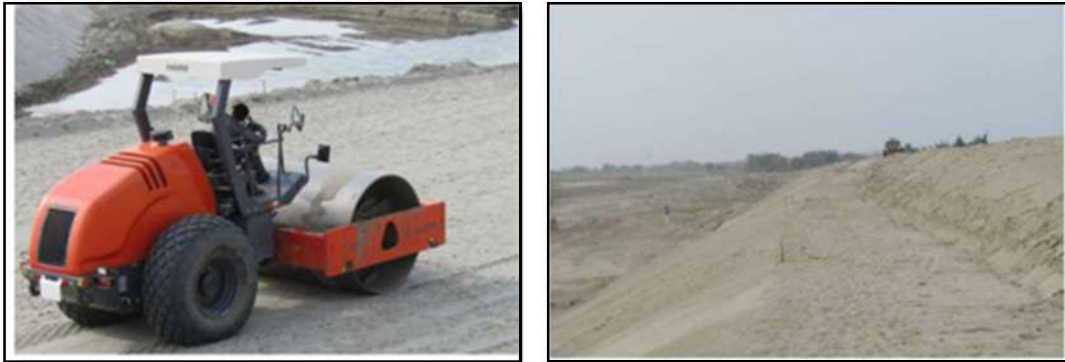
Fig. Preparation of subgrade before installation
