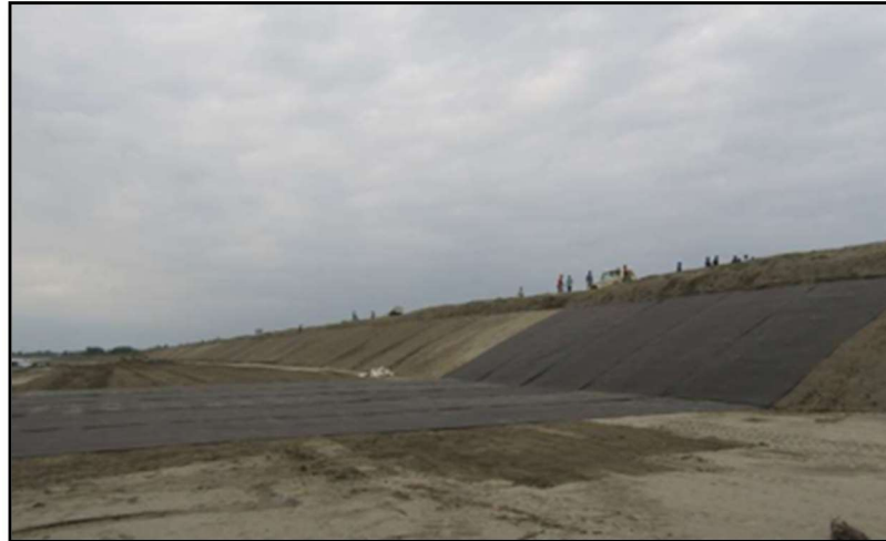
Fig. Laying of Geotextile layer
