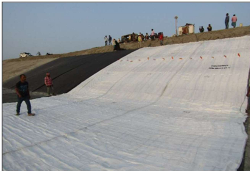
Fig. Laying of fabric
