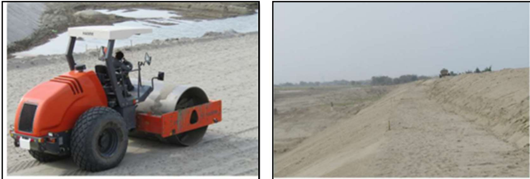
Fig. Preparation of subgrade before installation
