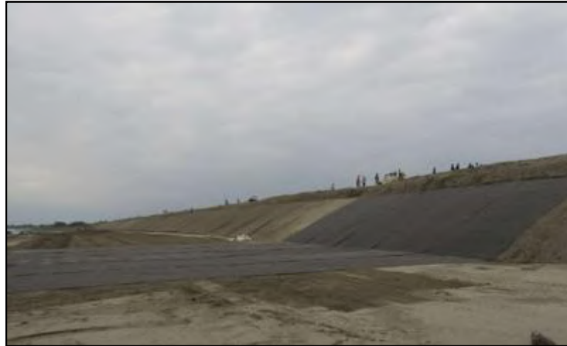
Fig. Laying of Geotextile layer
