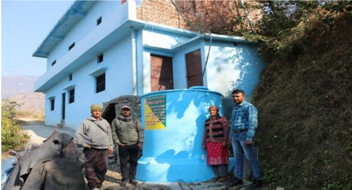
Fig: Construction of household roof rainwater harvesting tanks at Chamba, Tehri Garhwal
