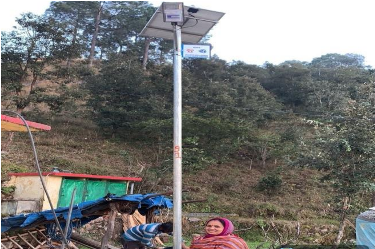
Fig: Installation of Solar Street light at Pratapnagar, Tehri Garhwal
