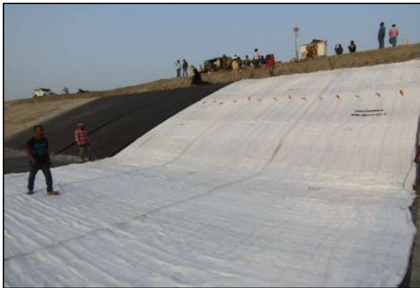
Fig. Laying of fabric
