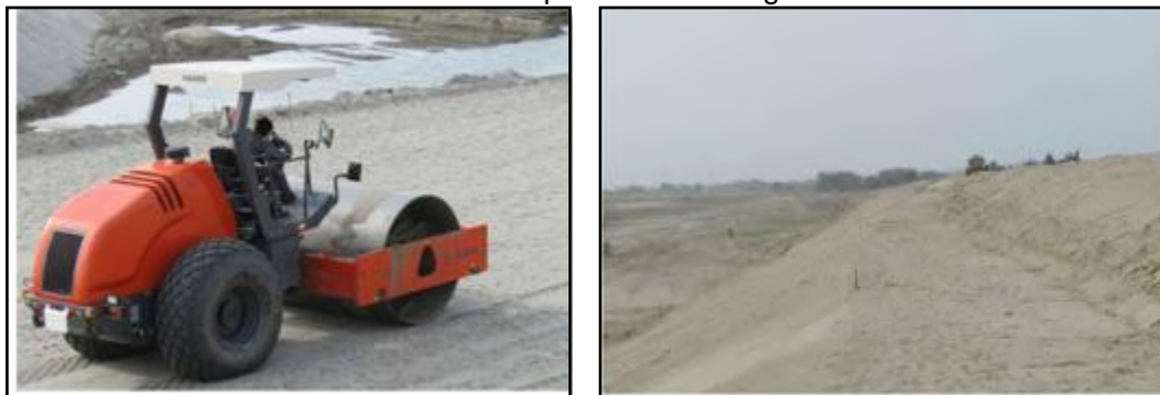
Fig. Preparation of subgrade before installation
