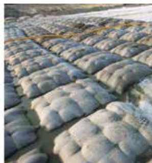
(b) Image showing installed Articulating Grouted Concrete Mattress after concrete filling
