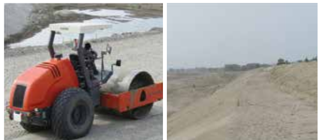
Fig.-3-Preparation of subgrade before installation
