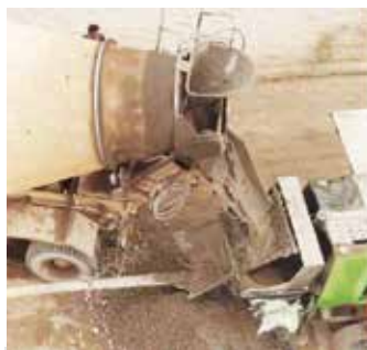
Fig.-6- (a) Image showing the process of concrete filling
