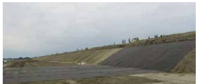
Fig.-4-Laying of Geotextile layer
