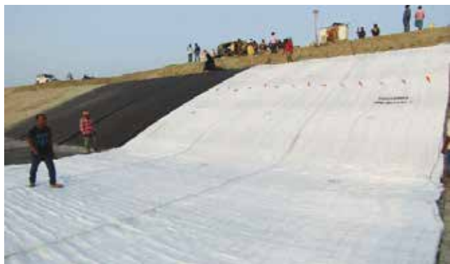
Fig.-5-Laying of fabric
