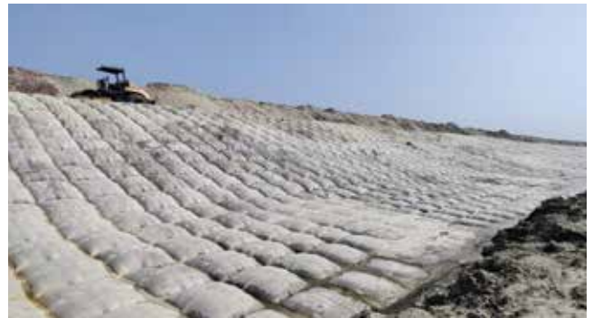
Fig.-2-Image showing installed Articulating Grouted Concrete Mattress over canal slope protection
