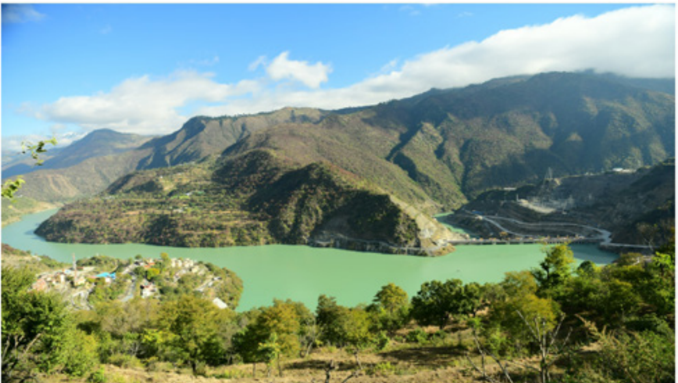
Upstream View of Koteswar HEP
