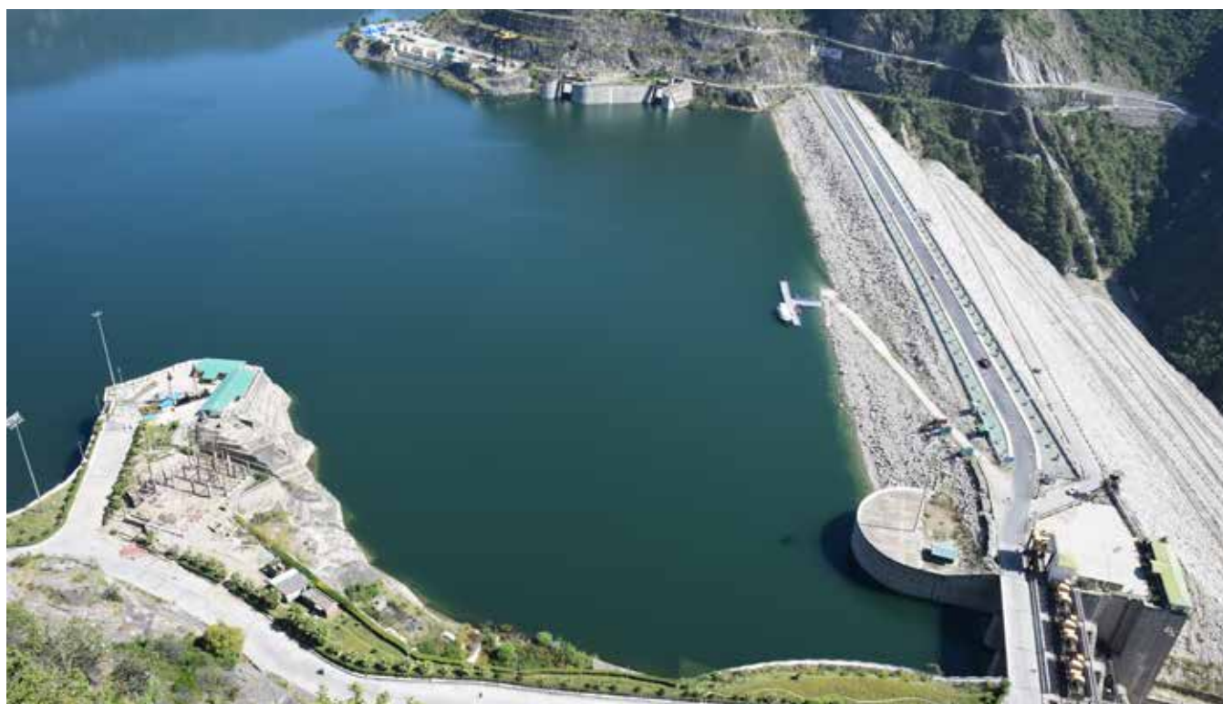
An overview of Tehri Dam & Reservoir
