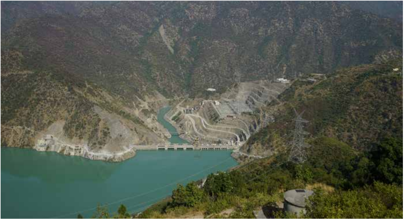
An overview of Koteshwar Dam & Reservoir
