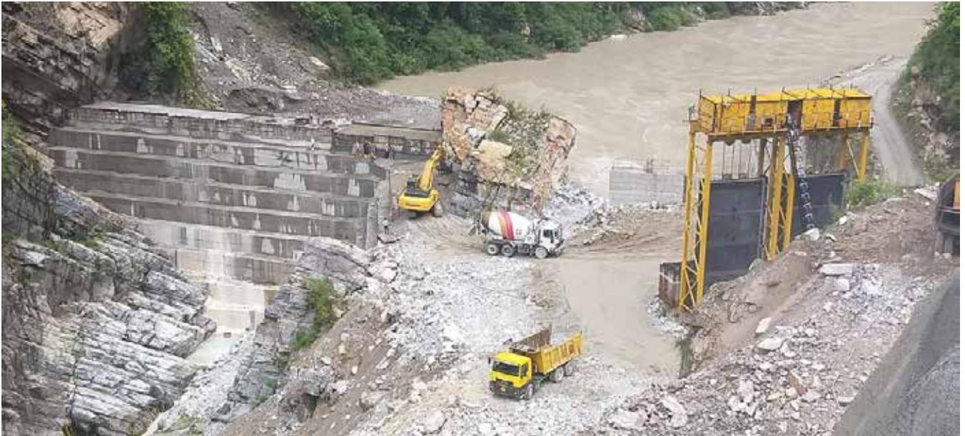
Coffer Dam of Vishnugad Pipalkoti HEP (444 MW), completed on 31.07.2019
