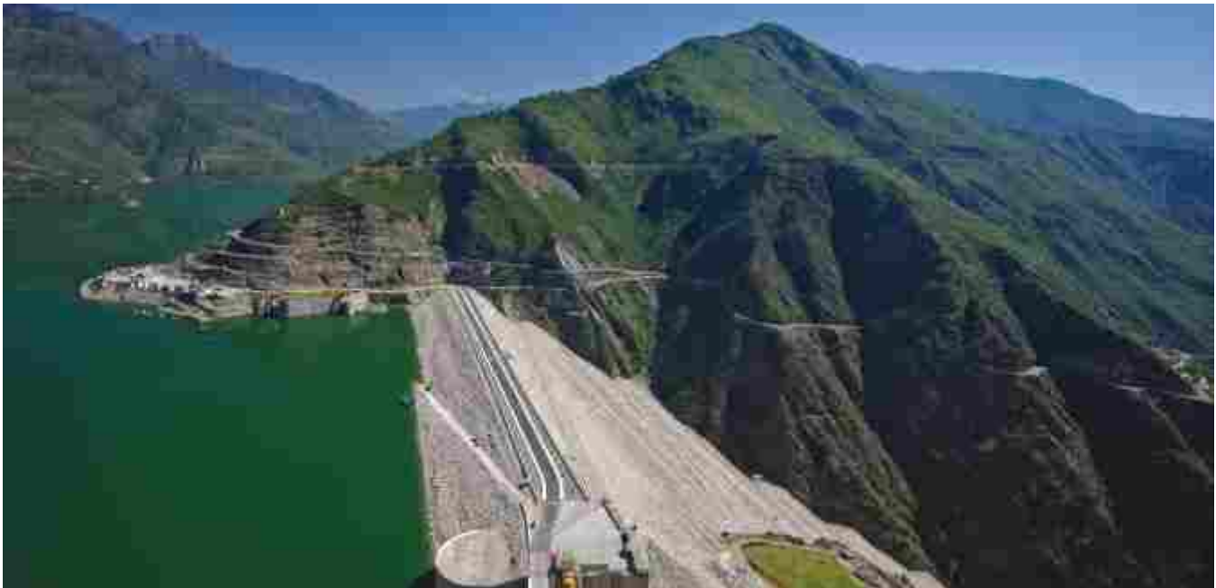
An overview of Tehri Dam & Reservoir
