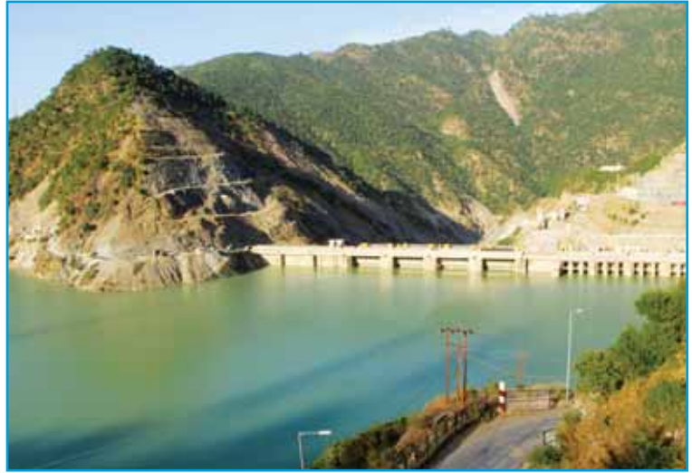
An overview of Koteswar Dam & Reservoir
