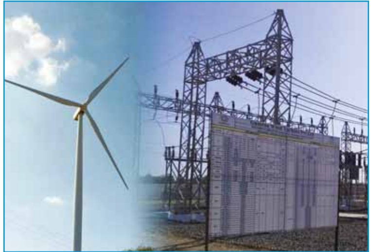
A view of Wind Power Project at Patan, Gujarat
