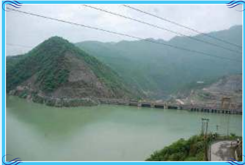
Upstream view of Koteswar Dam and Reservoir
