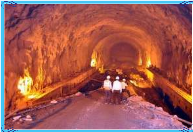
Underground Construction Work of Tehri PSP (1000 MW) in Progress
