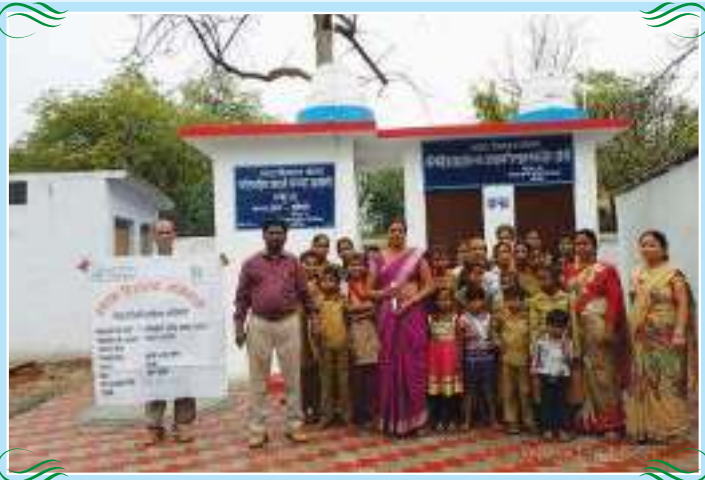
A View of Construction of Toilets in Govt. Schools under 'Swachh Bharat Abhiyan'
