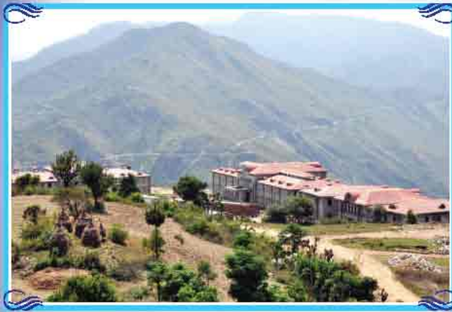
An overview of THDC Hydro Engineering College Campus at Tehri
