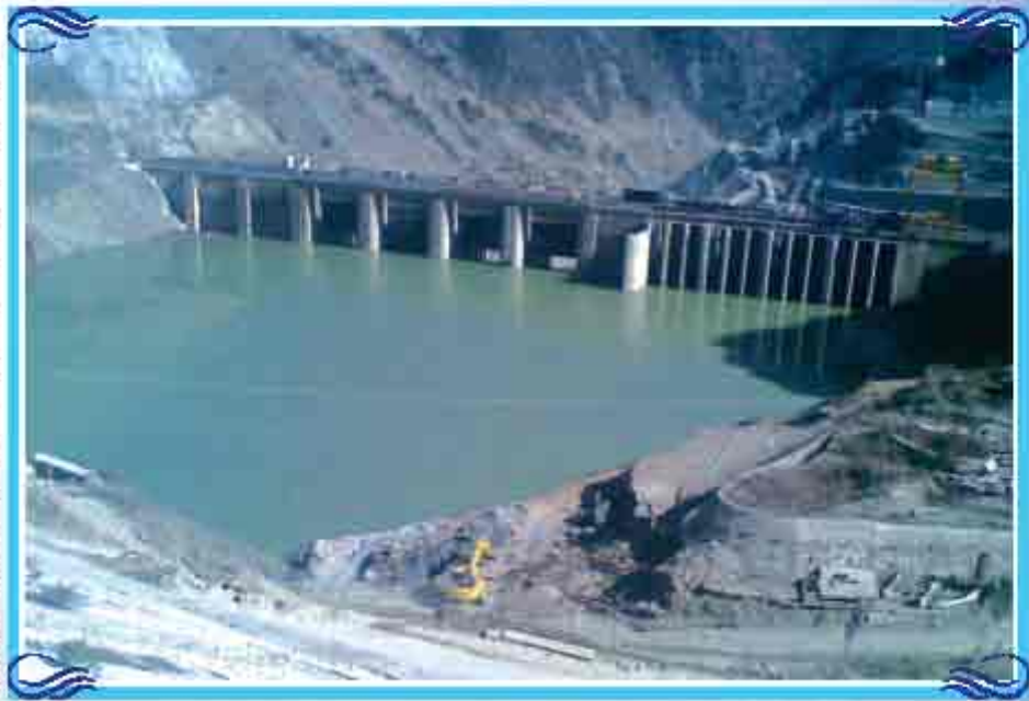
Up Stream view of Koteswar Dam
