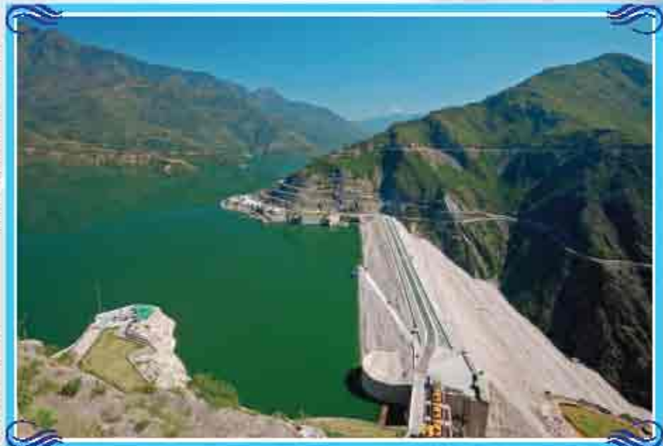
An overview of Tehri Dam & Reservoir
