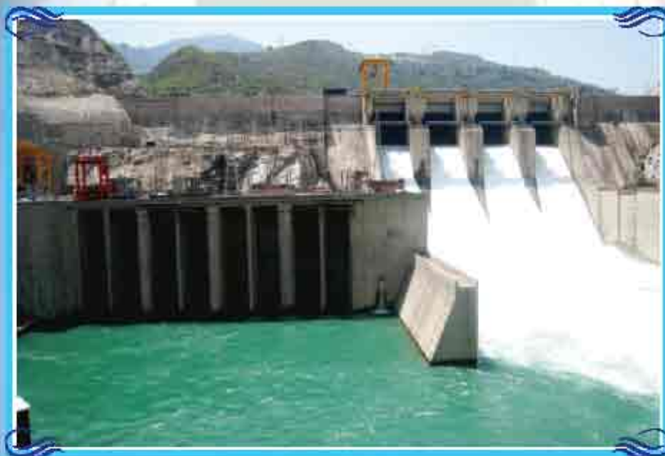
Down Stream view of Koteswar Dam
