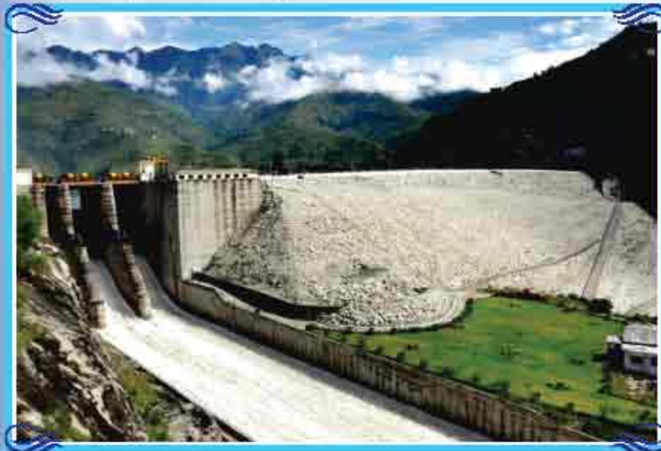
A view of Spillway of Tehri Dam
