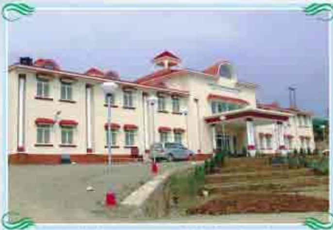
THDC Institute of Hydro Power Engineering and Technology at Bhagirathipuram, Tehri
