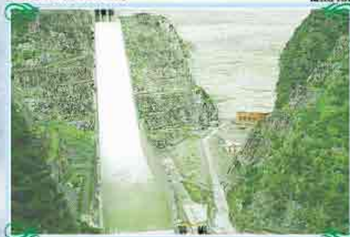
Spillway of Tehri Dam
