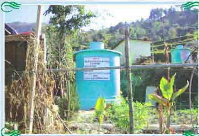
Rain Water Harvesting Tanks for water conservation at nearby Village of Tehri Dam Reservoir
