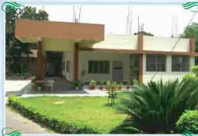
Building for Deaf and Dumb School at IIT Roorkee Campus developed by SEWA-THDC
