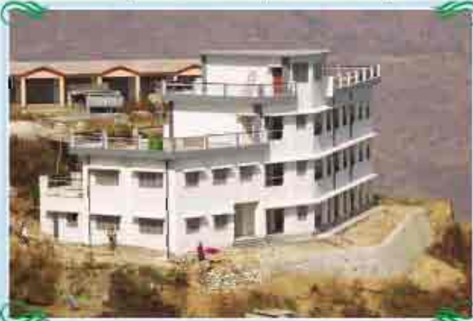
Building of Dr. Ambedkar SC/ST Hostel at New Tehri
