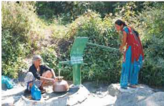
Installation of Hand Pumps at remote villages of Tehri District
