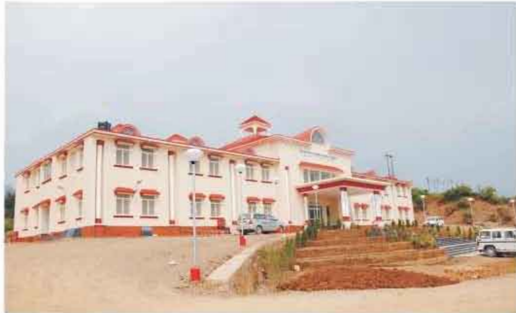
THDC Institute of Hydro Power Engineering and Technology at Bhagirathipuram, Tehri
