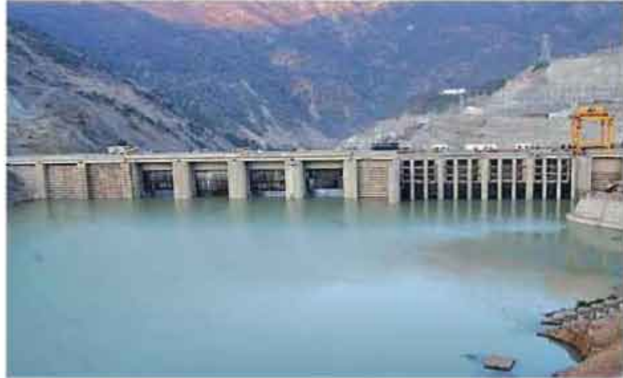
An overview of Koteswar Dam & Reservoir
