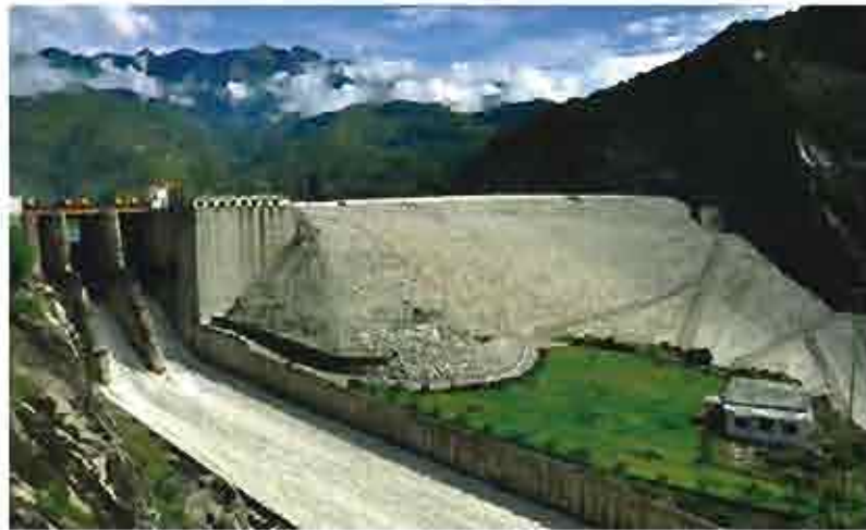
A view of Chute Spillway in operation at Tehri HEP
