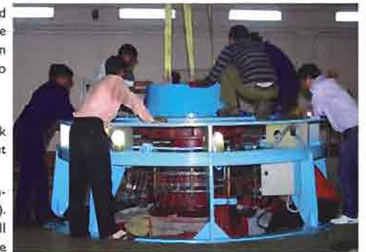
Assembly of Turbine Unit 400 MW at Koteshwar HEP
