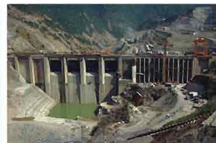
A view of work in progress in 400 MW Koteshwar HEP
