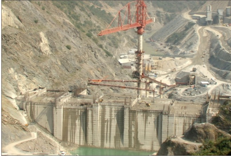
Work-in- progress at Koteswar HE Project.
