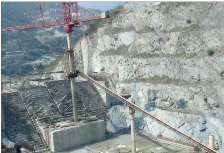
Work-in-progress at Koteswar HE Project
