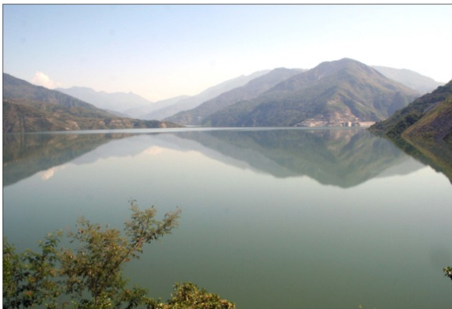
A Panoramic view of Tehri Reservoir
