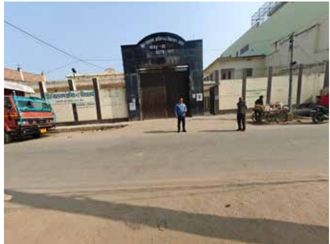
After: Boundary wall and gate constructed after demolition of the old hostel building
