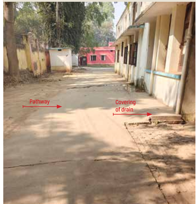
Pathway + Covering of drain
