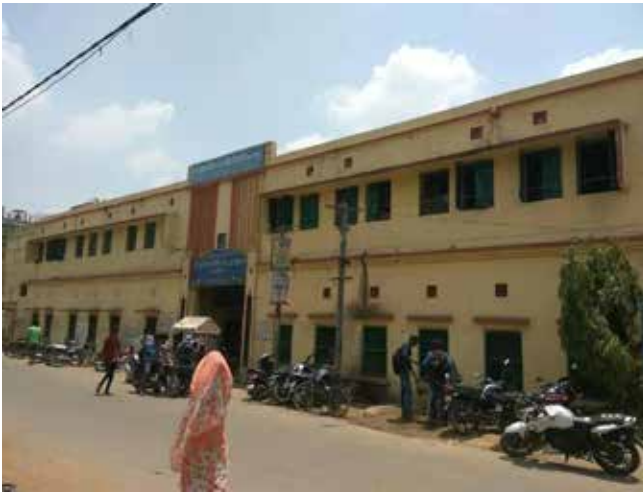
Before: the old hostel building abutting the main road
