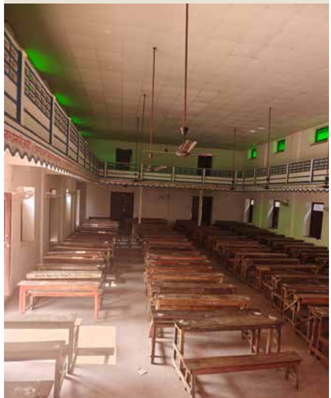
Seminar hall- tiling, false ceiling and fans provided under the project
