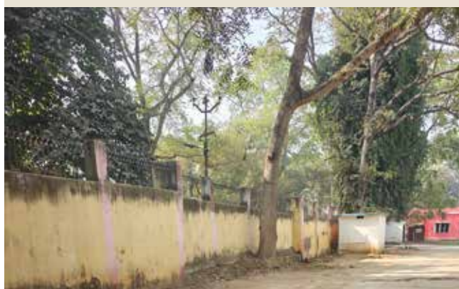
Boundary wall raised
