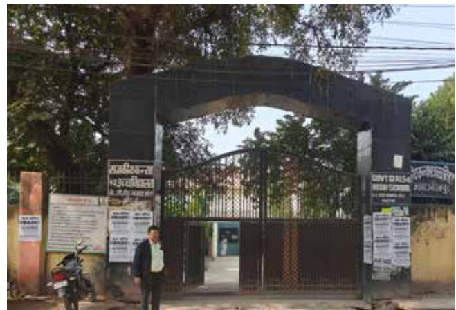
School gate constructed
