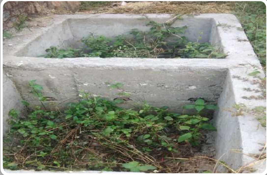
Non-functioning vermin compost pit at palam village
