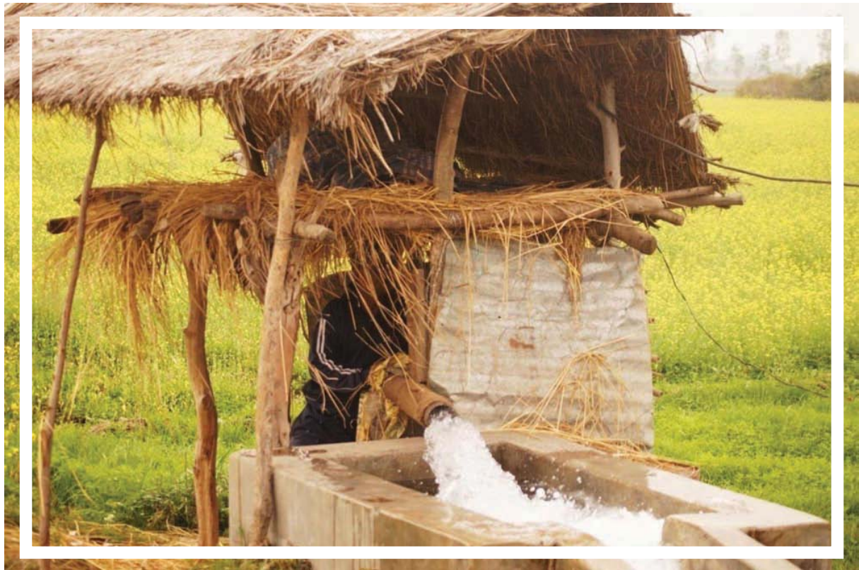
Figure 27: Tube well provided by THDC-SEWA to Farmer SHG
