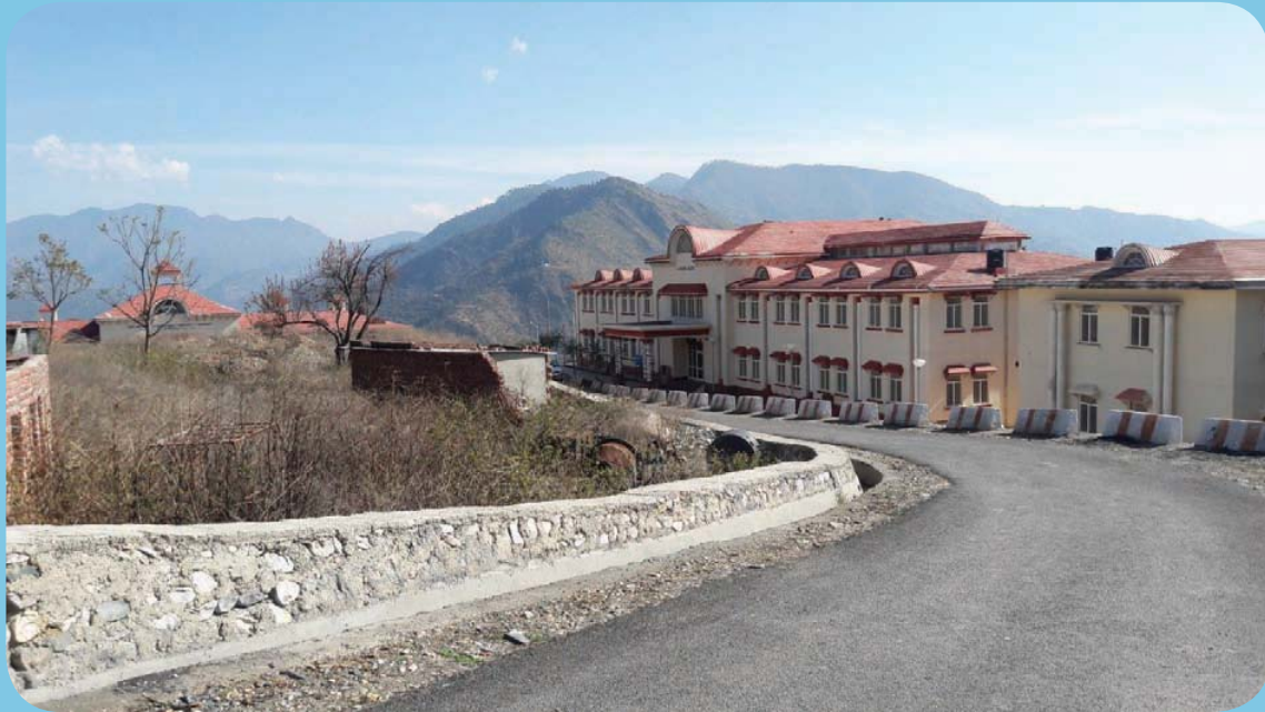
Figure 50: Engineering college block
