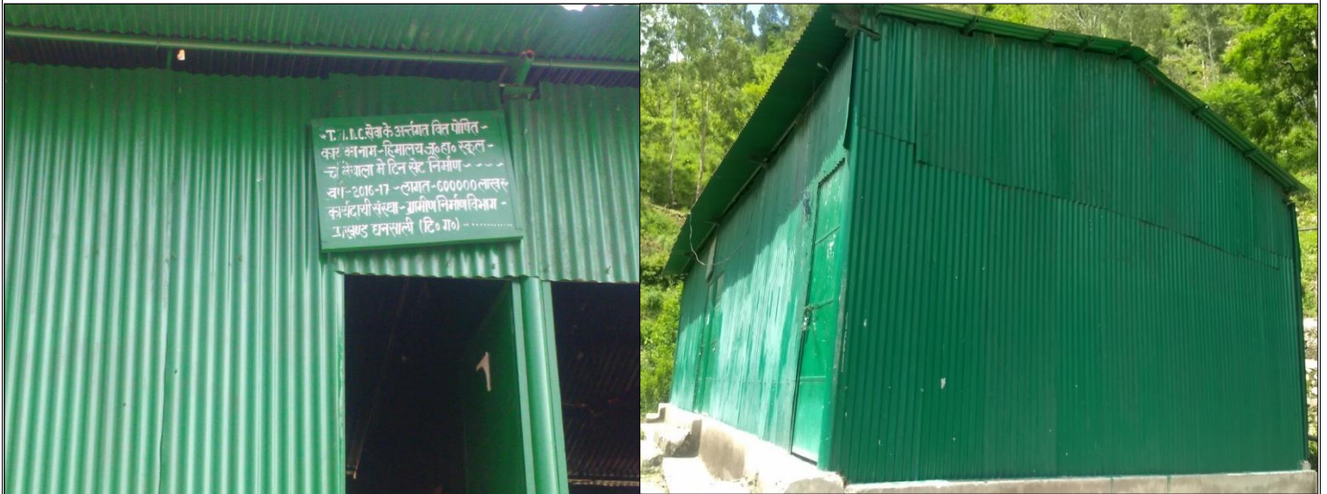
Tin Shed Classroom, Chamiyala
