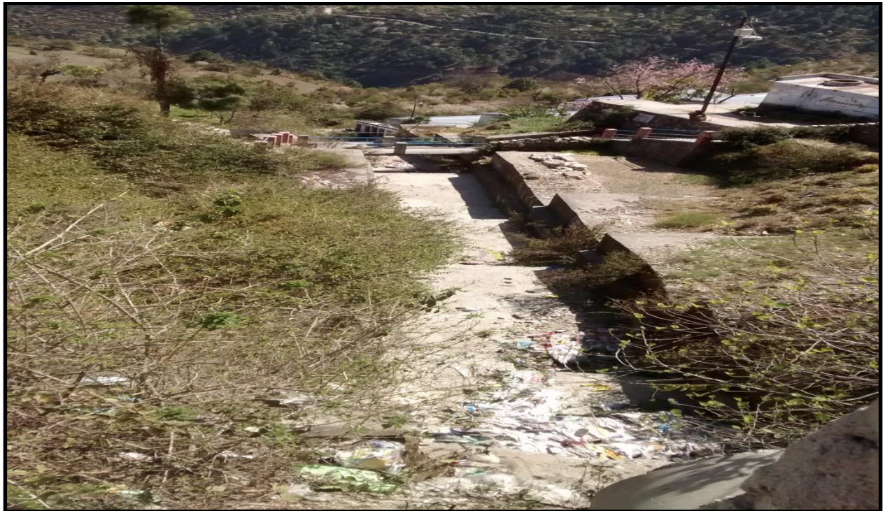
Picture 7: The nallah constructed for pipli
