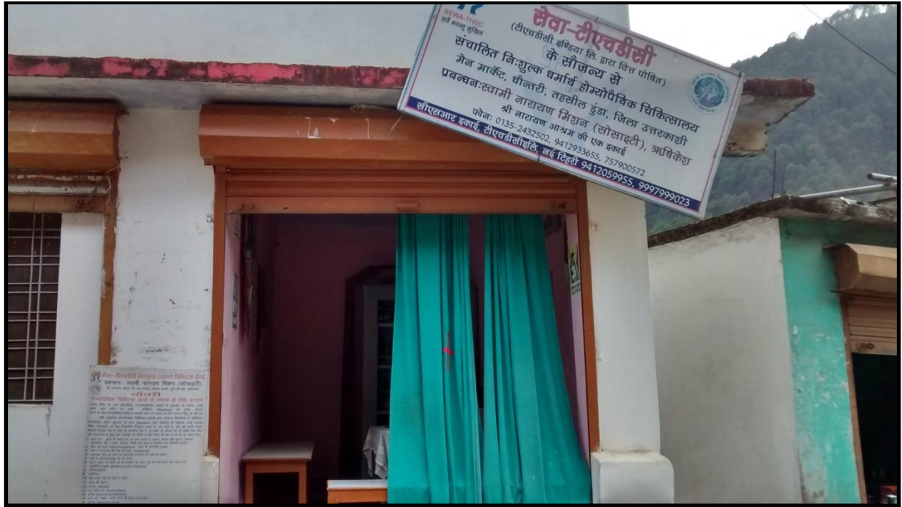
Picture 12: Dispensary constructed by THDC
