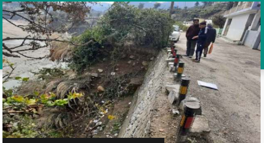
Constructed road wall in Chinyalisaur
