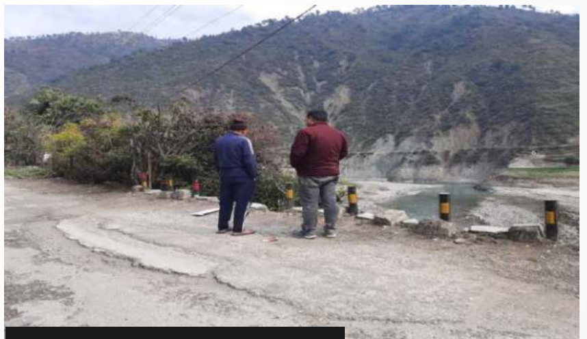
River view from the constructed road
