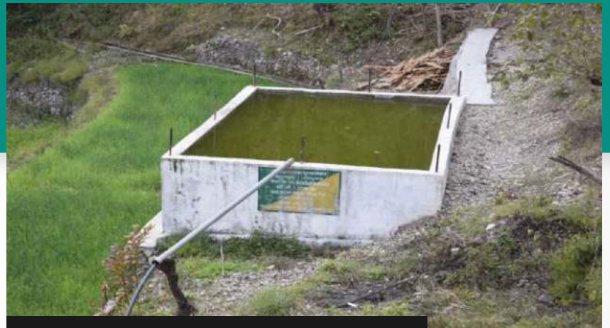
Irrigation tank with 38,520 liters capacity
