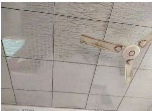
Figure 4.8 : False ceiling installed in the school
