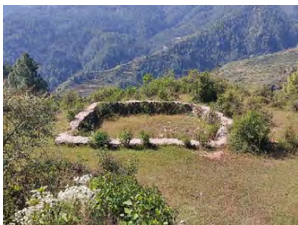
Figure 5.3 : Chal Khal constructed at project site
