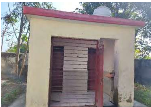
Figure 4.7 : Toilet constructed in the school
