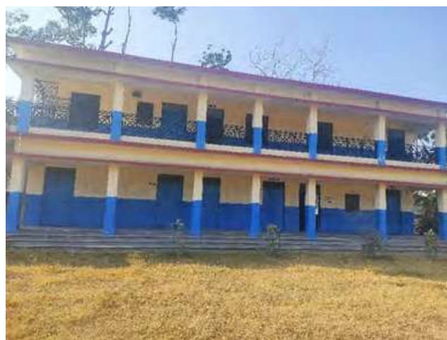
Figure 4.6 : Constructed laboratory on first floor of the building
