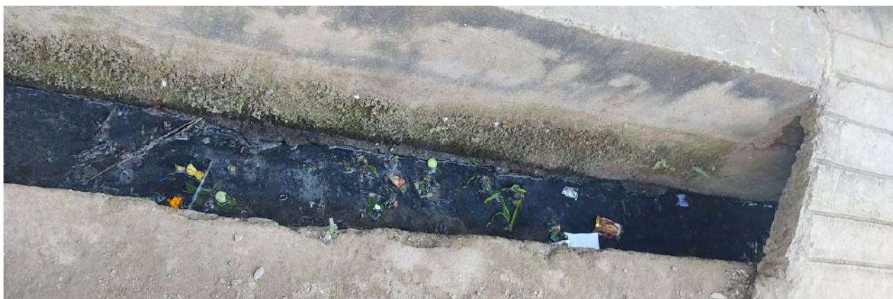
Figure 6.9 : Drain work in Meat Market, Indiranagar
