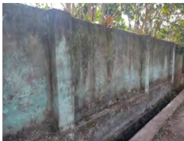
Figure 6.8 : Boundary wall-208 mtrs.
