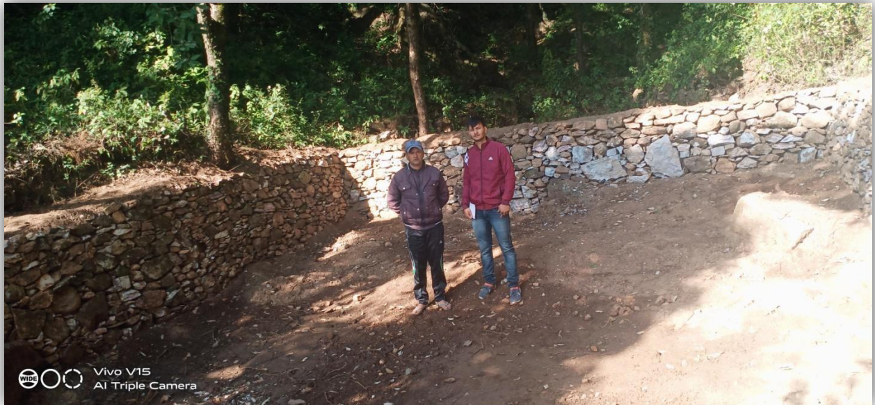
Final Stage Photo
