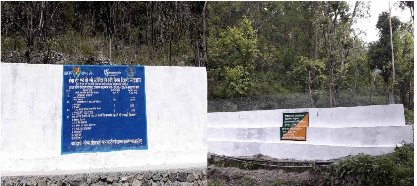
Inspection of LDPE Tanks and Irrigation Tank Construction by Agriculture Department, Tehri Garhwal
