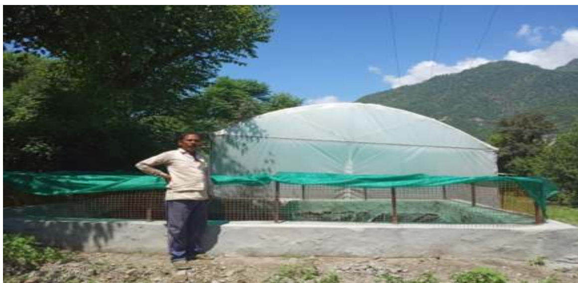
LDPE Tank Constructed in village Devri under ILEP
