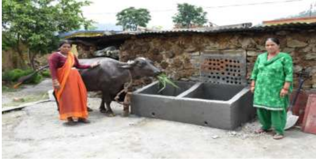
Construction of Mangers for Cattle under ILEP
