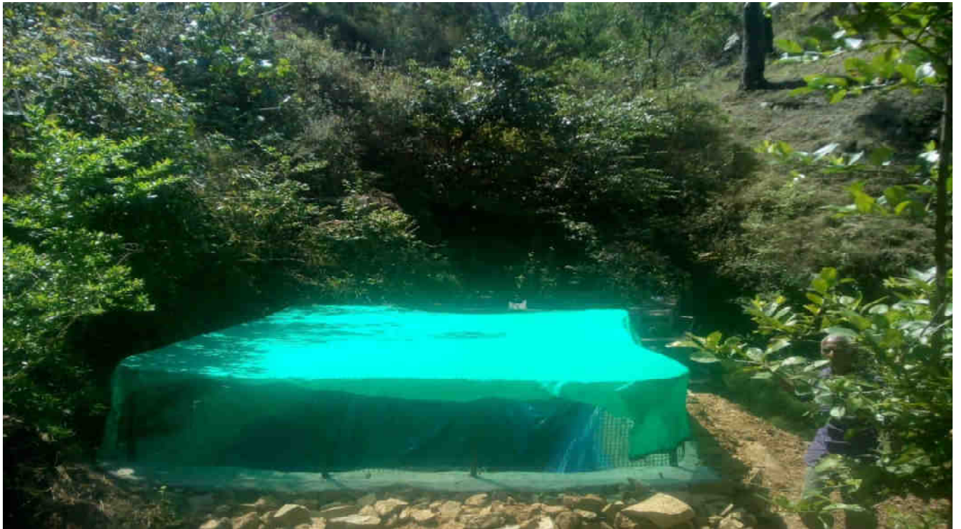
LDPE Tank Construction in Indrola Village under ILEP Project
