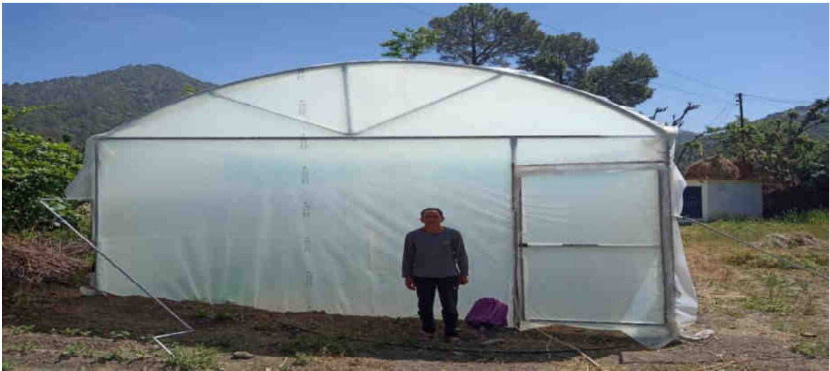
Poly House Construction under ILEP Project in Padagli Village
