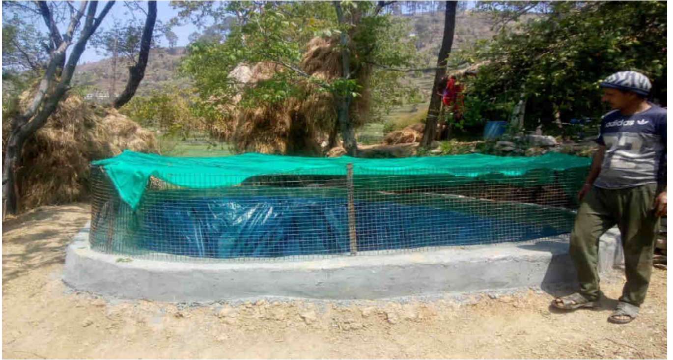
LDPE Tank Construction in Pilkhi Village under ILEP Project
