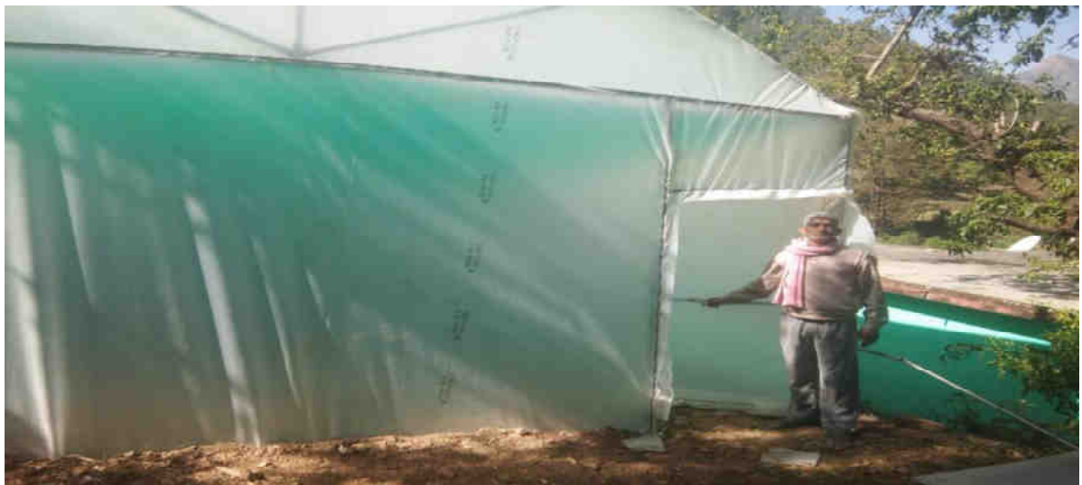
Poly House Construction under ILEP Project in Pilkhi Village
