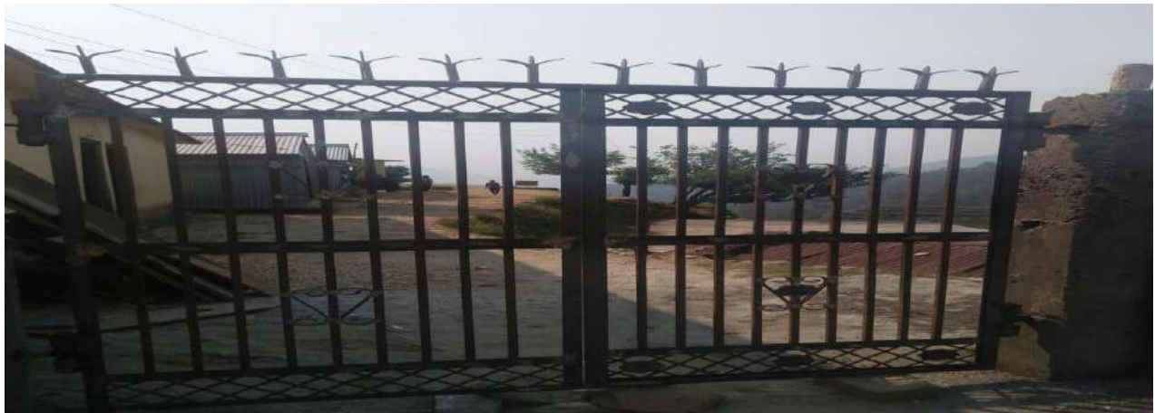
Renovation of School Gate
