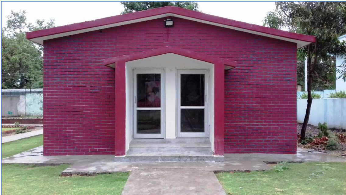
Toilet Block Front view
