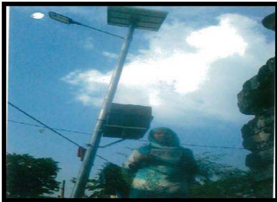
Solar lights installed at Bauradi Chawlk
