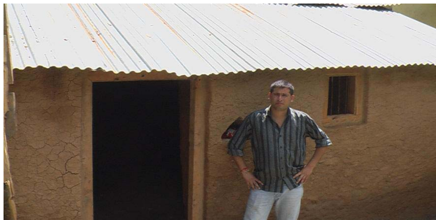
Eco hut under renovation
