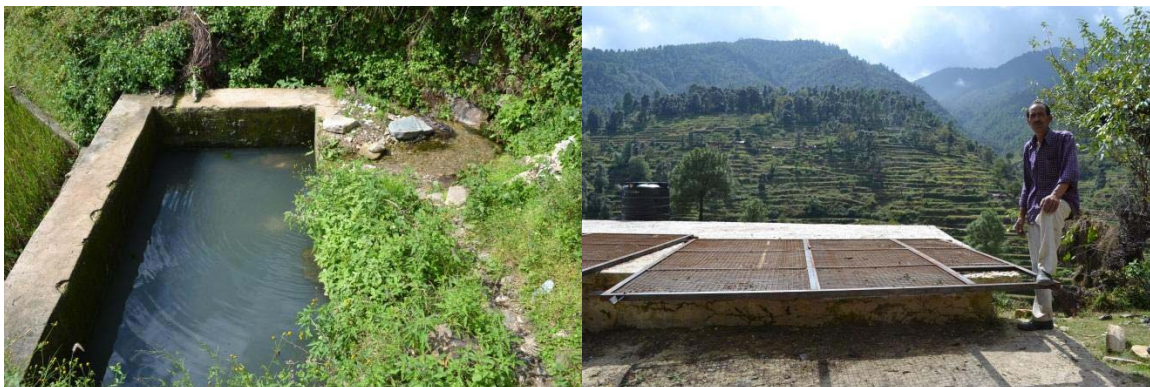
Construction of Fishry tanks
