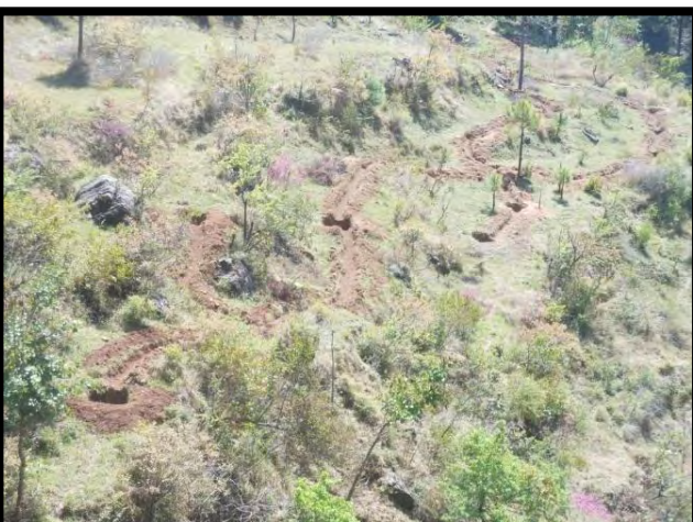
Recharge Pits with attached Trenches for rain water conservation
