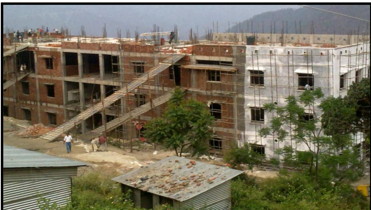
View of under construction Academic Block IV THDC-IHET, Tehri on 15.06.2014
