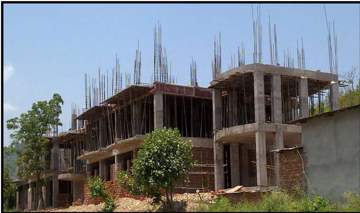
View of under construction Girls Hostel II THDC-IHET, Tehri on 15.06.2014
