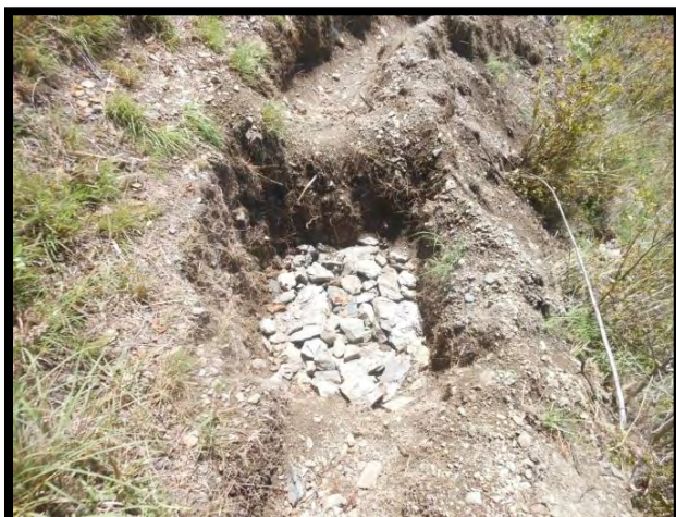
Recharge Pits with attached Trenches for rain water conservation
