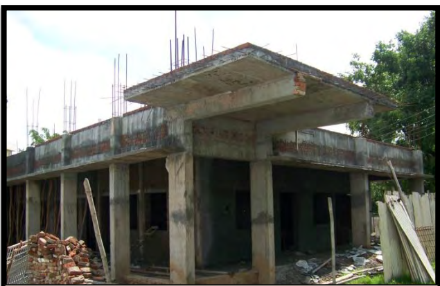
View of under construction deaf & dumb school building in IIT Roorkee
