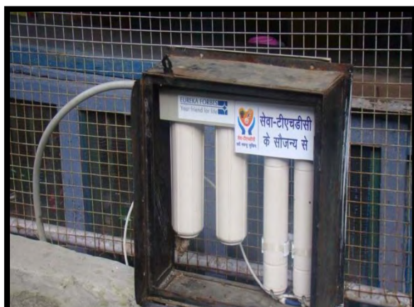
Providing & installation of water filters at Chamoli on 23.07.2012
