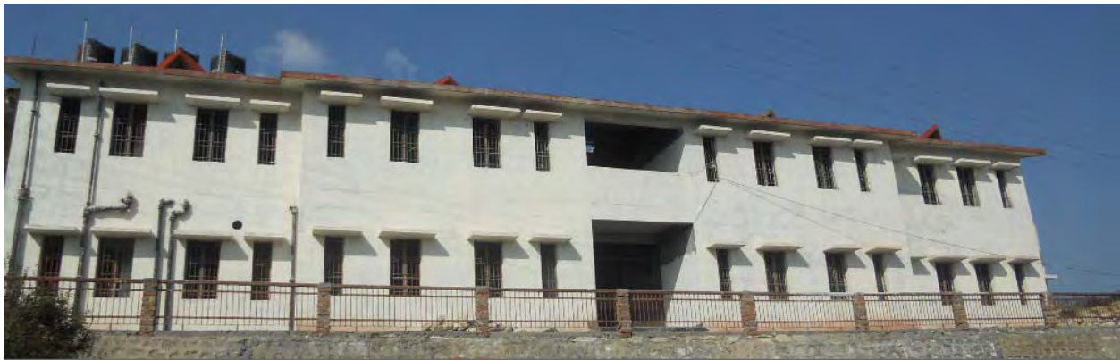
A view of under construction ITI Hostel at Chamba. Tehri
