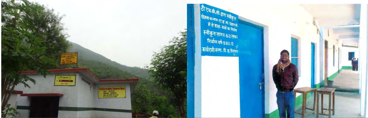
A view of constructed class room at Chopra (Jakhnidhar) & Ptagali (Bhilingana)
