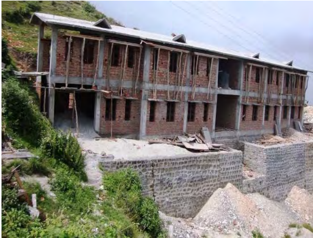
A view of under construction Boys Hostel at ITI, Chamba
