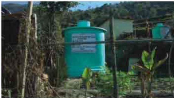
Water Harvesting installed by SEWA THDC at Kathuli village in Tehri an amount of ₹ 1.95 Cr. at New Tehri Town for the benefit of the students of SC/ST communities.
