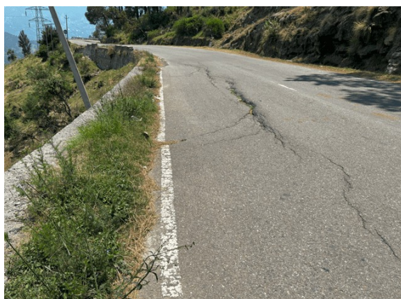
Fig.-7: Initial subsidence observed on the Road
