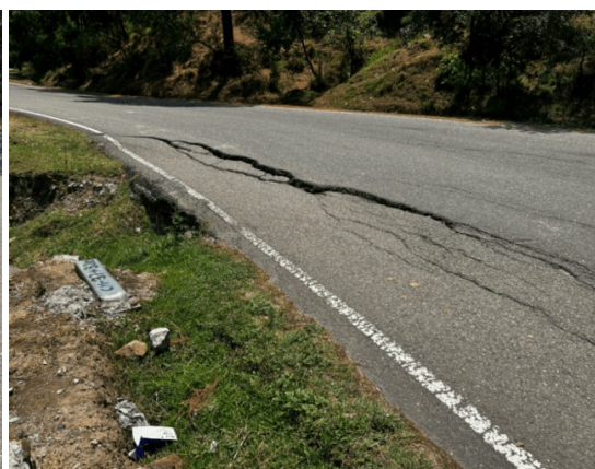
Fig.-8: Prominent Cracks developed on the pavement
