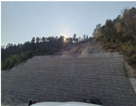
Fig.-6: RS wall with welded mesh facia under construction at Chinnyalisour, Uttarakhand along NH-34
