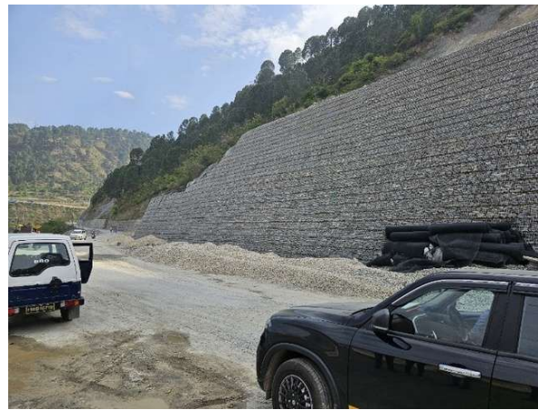
Fig.-6: RS wall with welded mesh facia under construction at Chinnyalisour, Uttarakhand along NH-34
