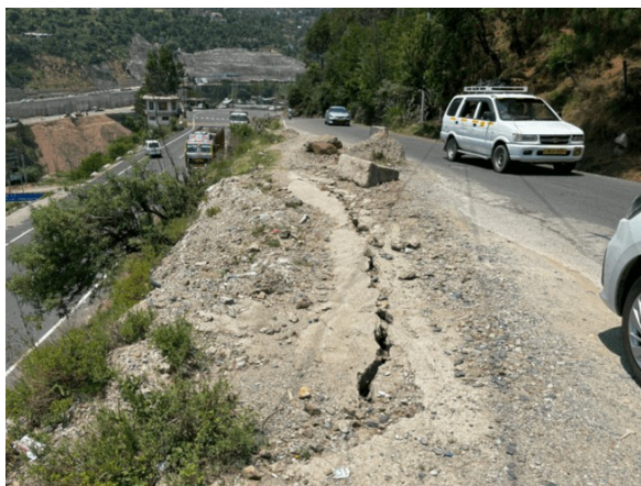
Fig.-9: Valley side movement of detached mass
