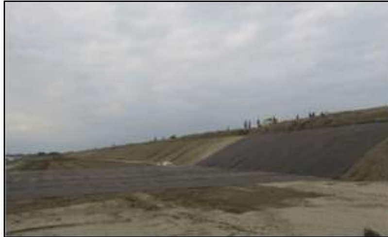
Fig. Laying of Geotextile layer
