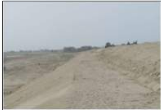
Fig. Preparation of subgrade before installation
