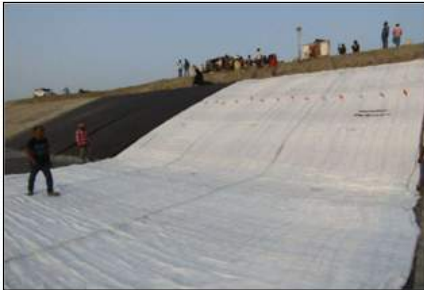
Fig. Laying of fabric
