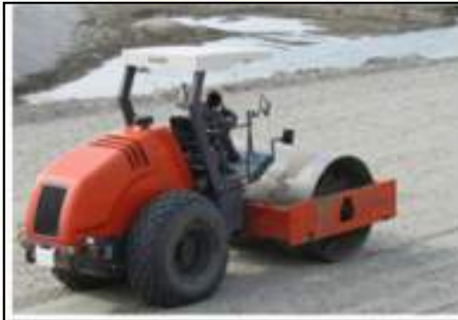
Fig. Preparation of subgrade before installation
