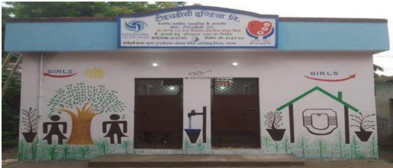
Fig: Construction of Community toilet at Govt. School, Bihar
