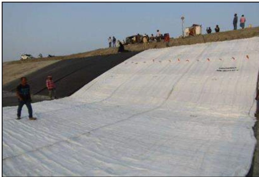
Fig. Laying of fabric
