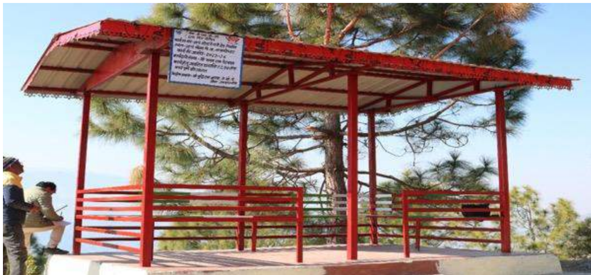
Fig: Construction of Yatrished at Thauldhar, Tehri Garhwal
