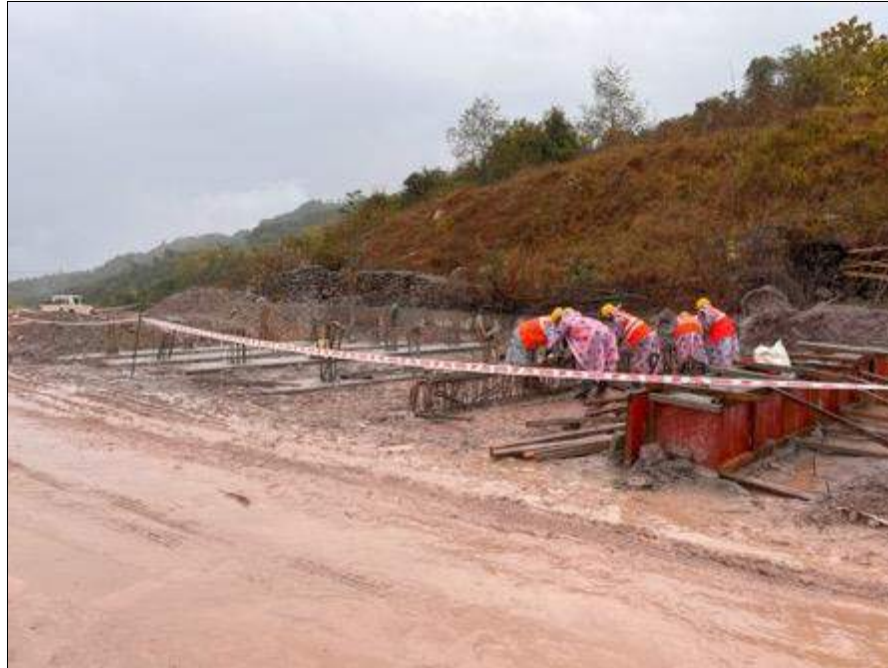
Fig. The proposed arrangement in construction at one of the site in Arunachal Pradesh along NH-513 (Pasighat-Yingkiong)
