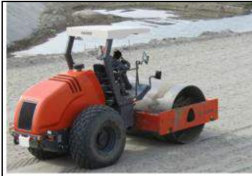
Fig. Preparation of subgrade before installation
