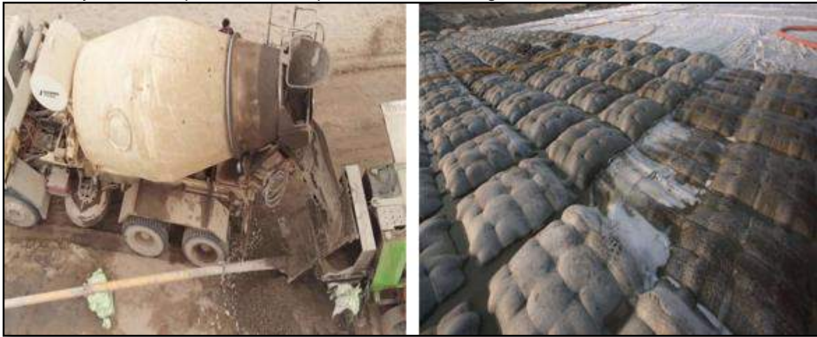
Fig.- (a) Image showing the process of concrete filling (b) Image showing installed Articulating Grouted Concrete Mattress after concrete filling
