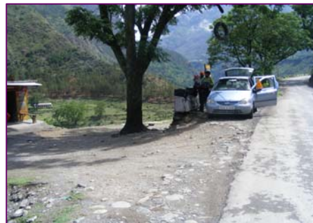
Starting point of approach road to Powerhouse & colony site
