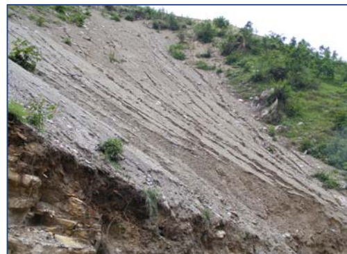
View Landslide in the project area
