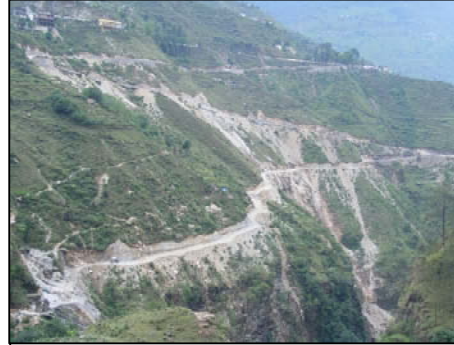
Approach Road to Maina Adit
