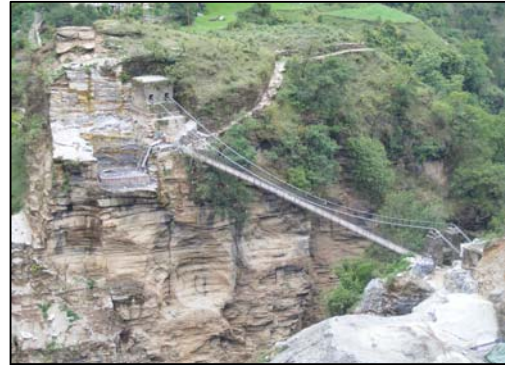
Bridge Construction on River Alaknanda , Approach road to Maina Adit
