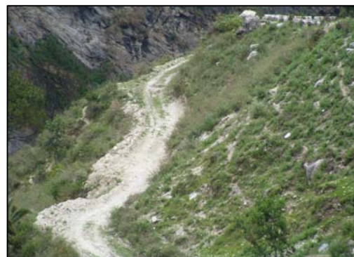
View of Approach Road (old road to Badrinath)
