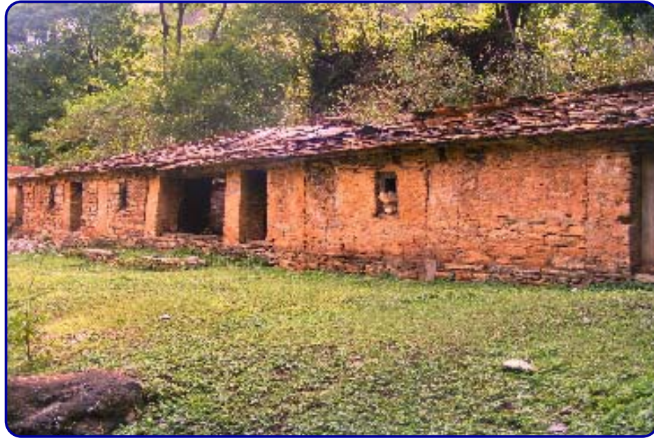
Figure-19 Abandoned shops (Heritage buildings) on Hat-Seasain ancient Route to Badrinath
