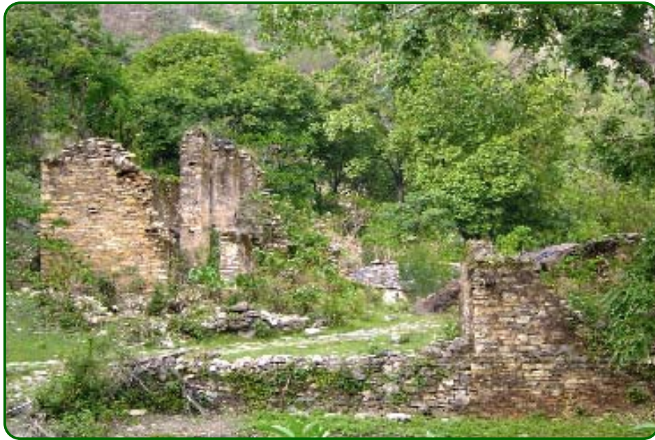
Figure-21 Remains of abandoned double storied guest house (Heritage building) on Hat- Seasain ancient route
