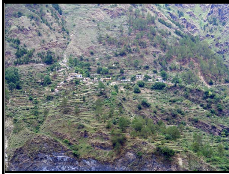
Figure-56 General view of the Dwing village
