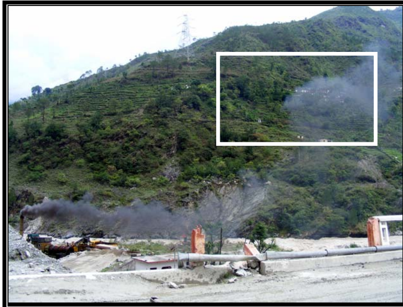
Figure-69 General view of the Durgapur village
