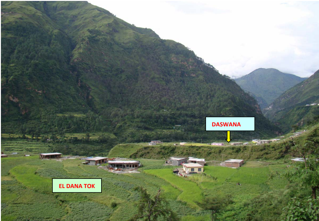
A VIEW OF HAAT RELOCATION SITES
