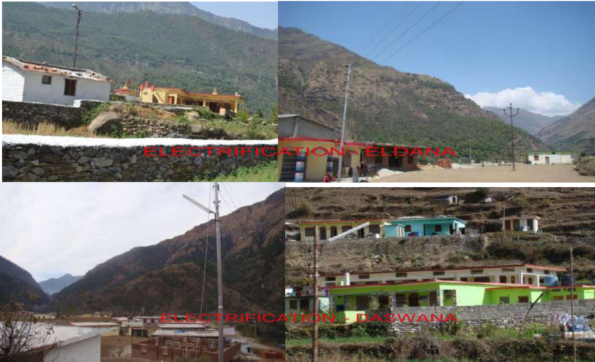
Electrification work in villages Eldana & Daswana
